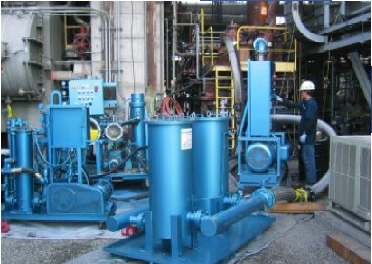
Flushing rig set up to clean the system
