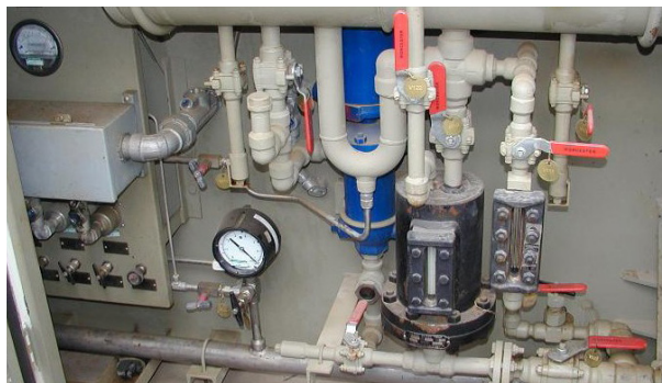
Fig. 1 - Controls for a hydrogen seal system in a large frame gas turbine.
