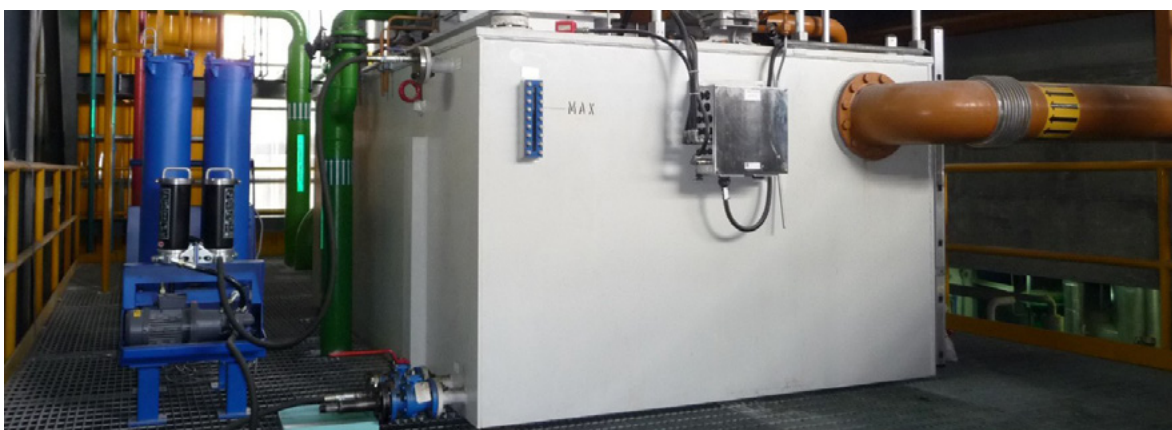
Fig. 7 – Fluitec ESP Varnish Mitigation System installed on a turbine.
